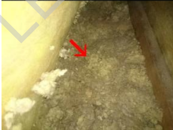
Loose fill insulation
