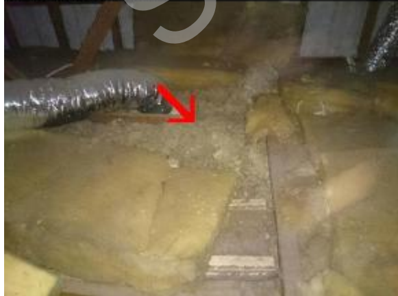
Partly installed batts
