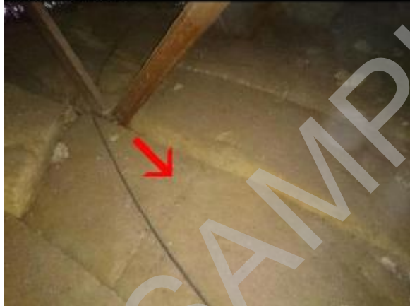
Partly installed batts
