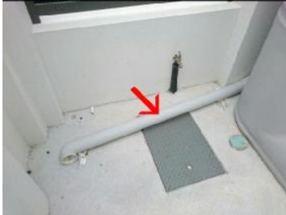
Removed overflow pipe to tank
